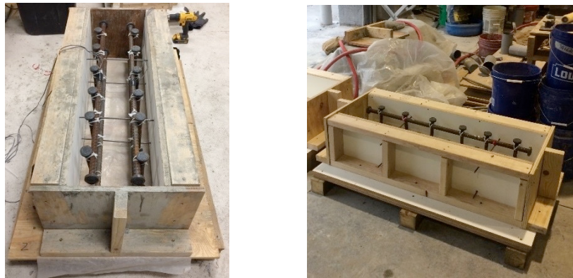
Figure 3.3: Rebar Placement Prior to Casting (Malone 2019)
